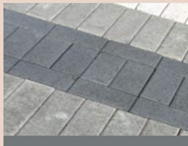
Concrete block production
