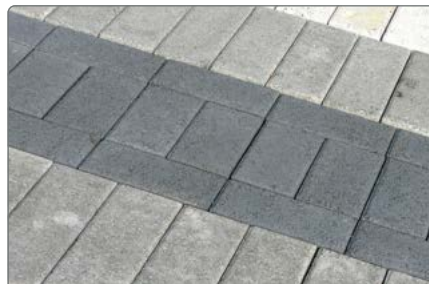
Concrete block production
