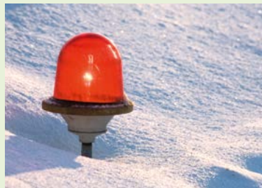
Snow removal at airports
